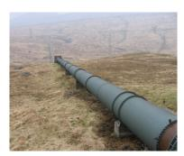
Line pipe is the type of pipe that is used in the surface transmission of oil, natural gas and other fluids.
